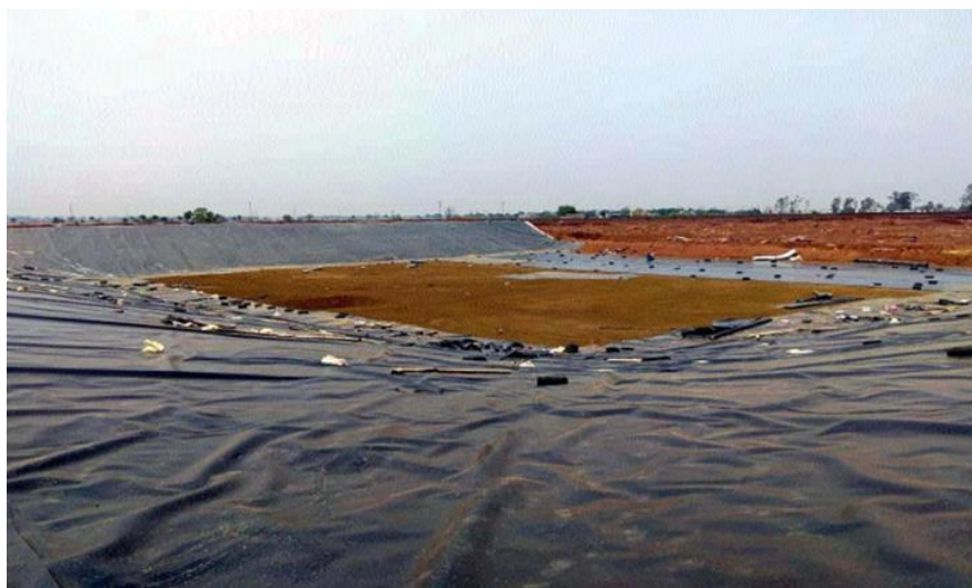
Figure 4.3: Sarona Trenching Ground at Raipur.
